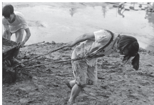
010 Construction of the Beijing University swimming pool by students, June 1958. © Fondation Henri Cartier-Bresson / Magnum Photos
