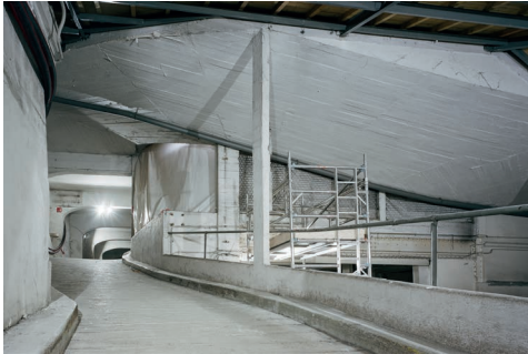
013 Fondation HCB, 79 rue des Archives, February 2017 Vehicle access ramp to the upper levels of the old car park that was destroyed at the request of the architects of Les Bâtiments de France to recreate the 18th century courtyard. © Cyrille Weiner
